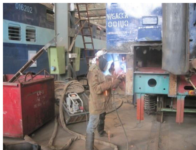
Fig 5: Welding work at End Panel
