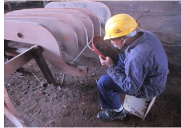
Fig 9: Swan neck weld repairs
