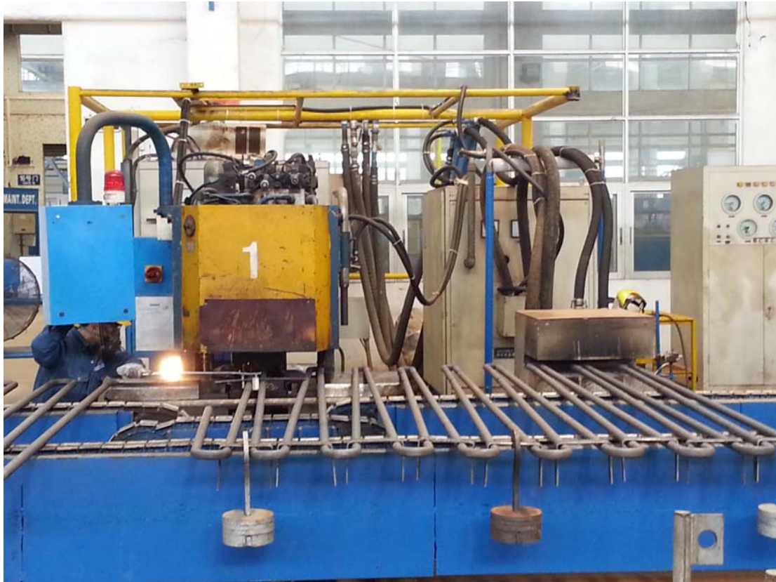
Medium-Frequency Induction Furnace used in Coil bending from “1.5-D” to “1-D” [W.H. Tsang]
