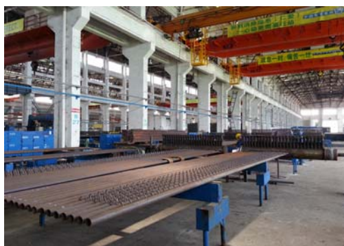
Stud welded on tubes to grab refractory standards. [W.H. Tsang]
