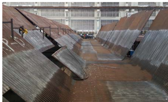
Wall Panel in full final length assembled for Duke Energy project [W.H. Tsang]
